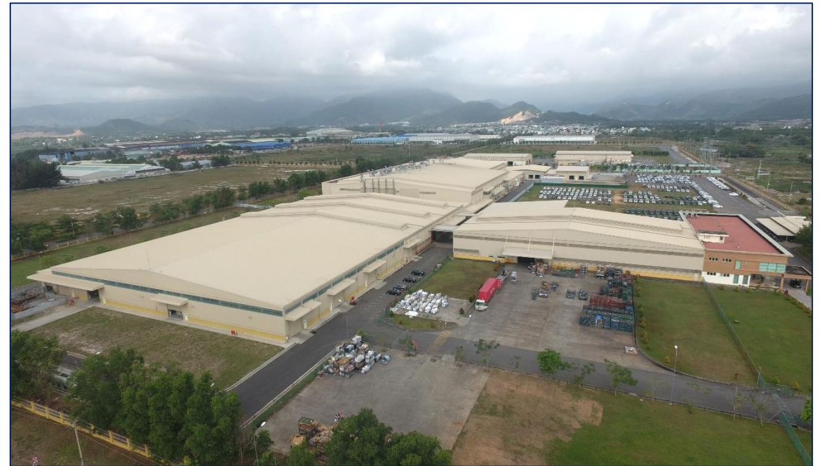
Plant Expansion in Danang, Vietnam
