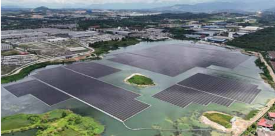
In January 2024, the Group's first floating LSSPV plant in Serendah, Selangor successfully commenced operation.
