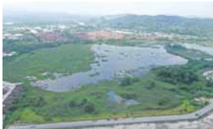
The Lake at the site of the project, heavy vegetation before site clearance.
