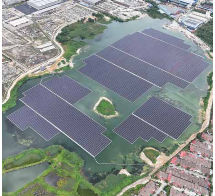
LSSPV – Serendah is an important milestone signifying the Group's first venture into the renewable and sustainable energy sector.
