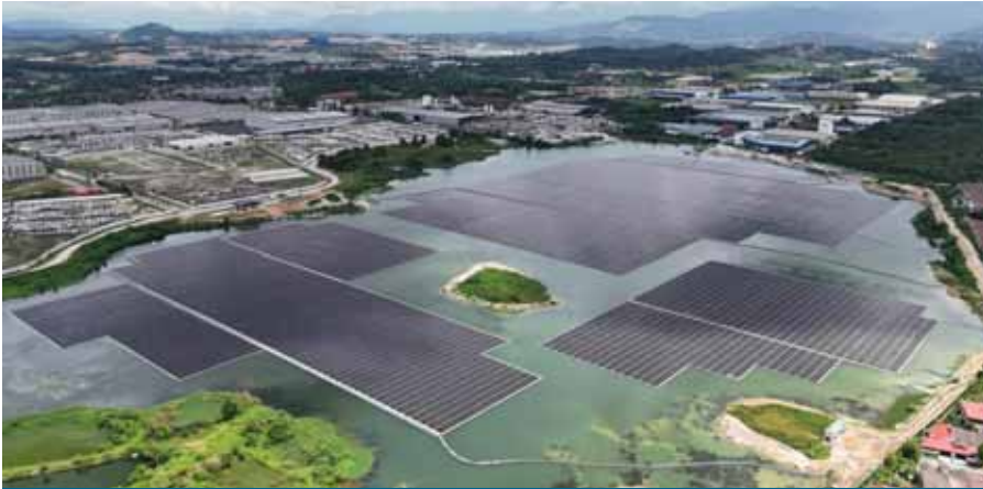
In January 2024, the Group's first floating LSSPV plant in Serendah, Selangor successfully commenced operation.
